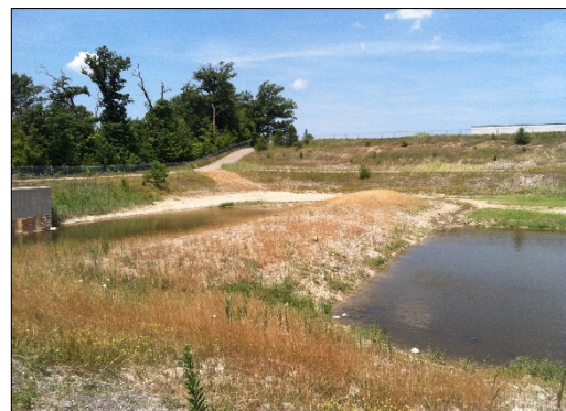
North Detention Basin after 2012 Retrofit
