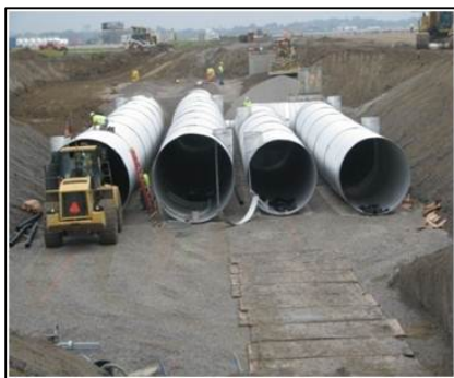
Underground Stormwater Management Facility Under Construction
