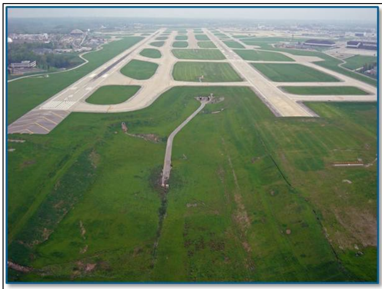
Central Detention Basin
