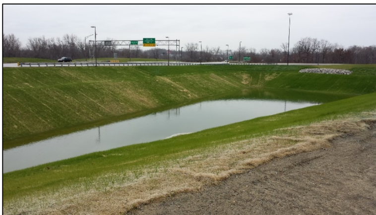
South Retention Basin (Photograph Taken 11/21/2013)
