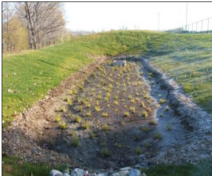
Riveredge Bioretention Cell
