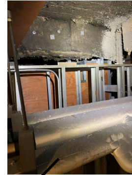
Ceiling; crossbeams; hot-water pipes
